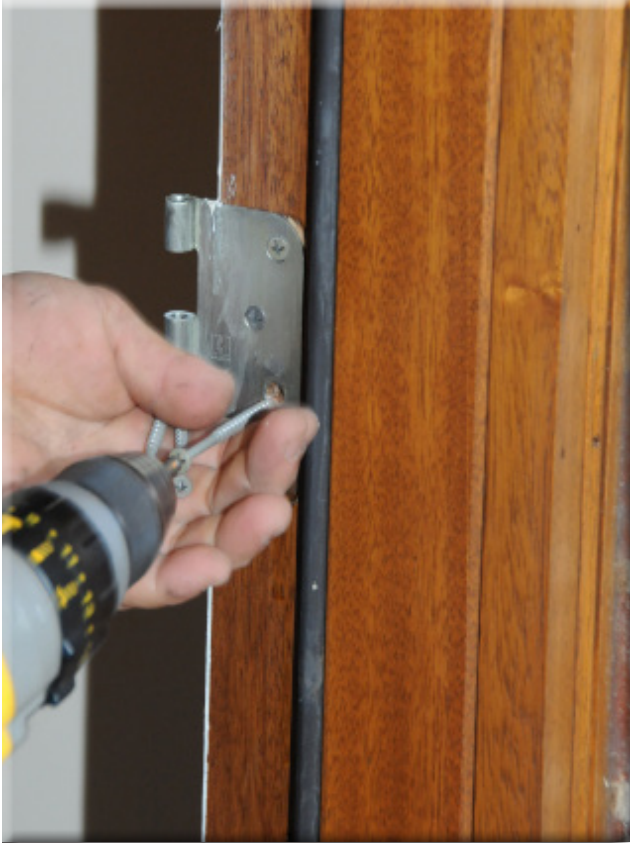
Figure 1.4- These screws go through the jamb and into the surrounding framework. They must be removed before proceeding to the next step.
