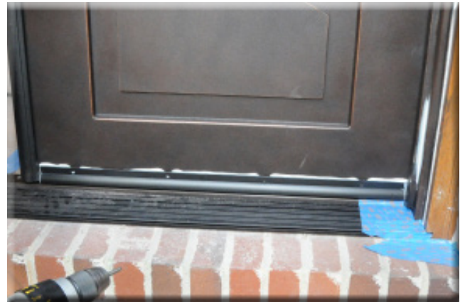
Figure 2.17- The sweep is in place. The caulk can easily be cleaned off the door.
