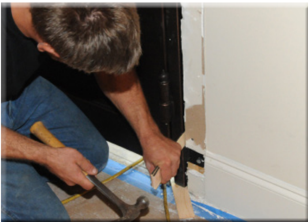
Figure 2.12.3—Keep working on the shimming. The door will eventually line up.
