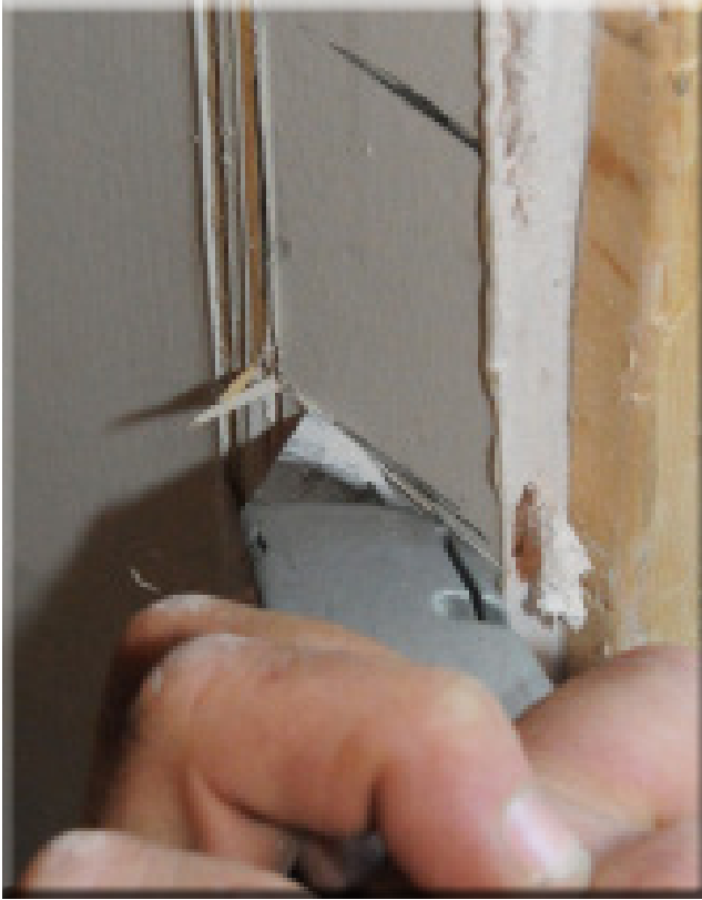
Figure 2.3- Make several passes through the wall board with the utility knife. Alternatively, you may want to use a router for this step. Just be careful not to remove any material from the studs.
