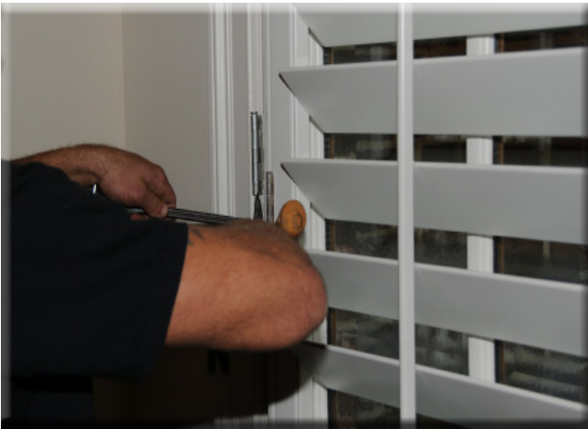
Figure 1.1- Removing pins from existing door.
