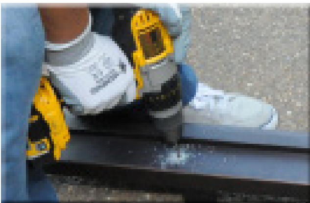
Figure 2.4.1- Position the hole for the alarm contact so that it is towards the center of jamb space that will be occupied by the active door.
