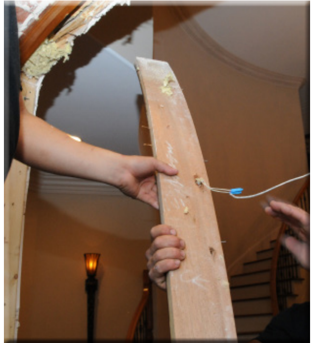
Figure 1.9- The alarm contact wire needs to be disconnected and installed in the new jamb.
