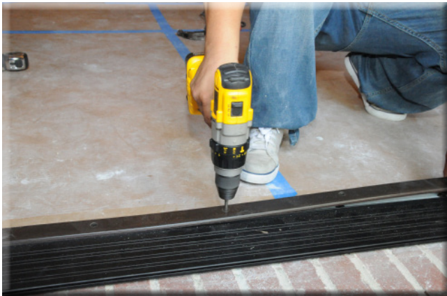
Figure 2.14.1- Loosen each screw a little at a time so as not to damage the riser of the threshold.
