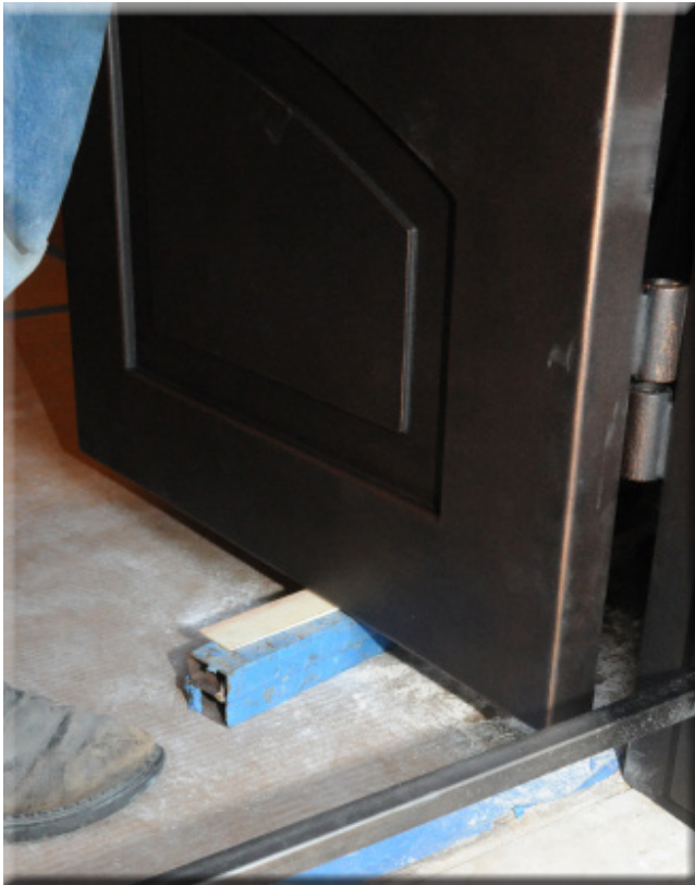
Figure 2.9- The door hinge barrel is directly above the jamb hinge barrel. There is a space of about 1/2" which will allow for placement of the washer.
