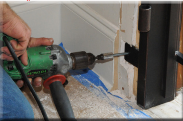
Figure 2.7.1- Secure the jamb with 5/16" x 3" lag screw at the bottom first.
