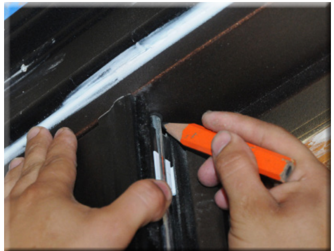
Figure 2.15.1- Make sure to apply pressure to the door while marking the top flush bolt position.
