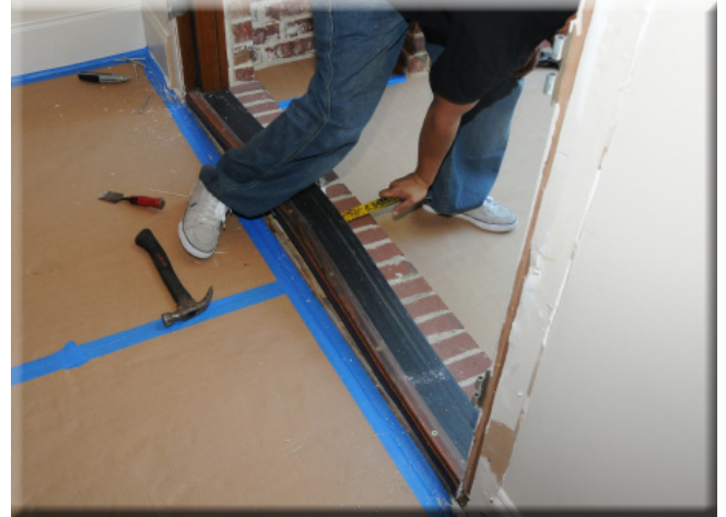
Figure 1.5.1- Break loose the threshold from the concrete. This may take some force as you will be prying against glue and screws.
