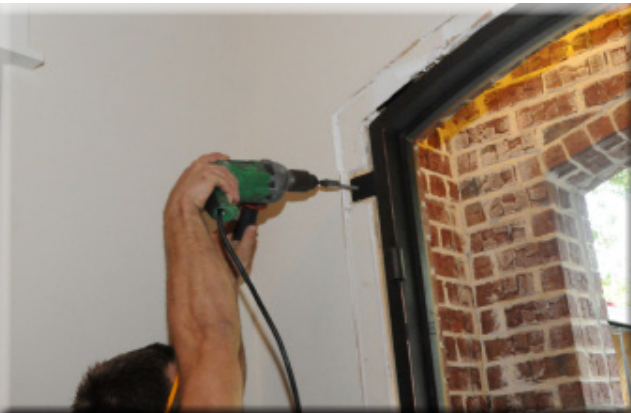
Figure 2.7.2- Screw in the top side brackets. Only four screws will be used to hold up the jamb until door is fully adjusted.
