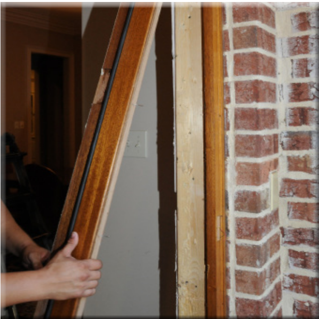
Figure 1.8- The jamb components are being removed while preserving the exterior brick mold.
