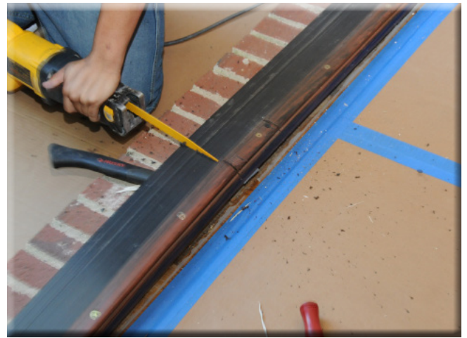
Figure 1.5.2- Cutting the threshold will help in its removal. A reciprocating saw is ideal for this. A circular saw will work nicely as well.
