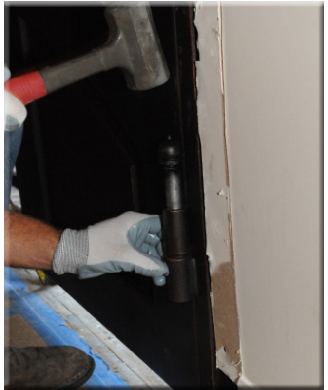
Figure 2.11- The hinge pins may need some help seating. A rubber mallet will apply enough force without damaging the paint.
