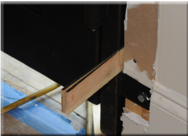
Figure 2.12.2—Loosen the lag screw a bit so that the door jamb can move when you are driving in the shims.
