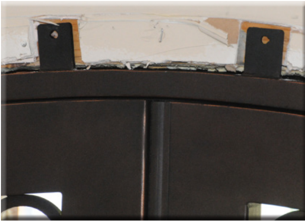
Figure 2.12.1—These doors do not quite line up at top. The right door is slightly lower than the left door. Shimming at the lower right of the door should push the right door up.
