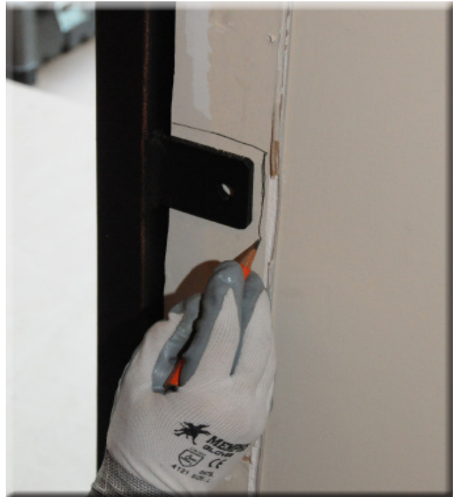
Figure 2.2- Trace the tab out about 1/2" more all the way around. Be careful not to mark beyond the old caulk line. You do not want to remove the wallboard beyond that line. If you do, the trimwork will not cover it up completely.
