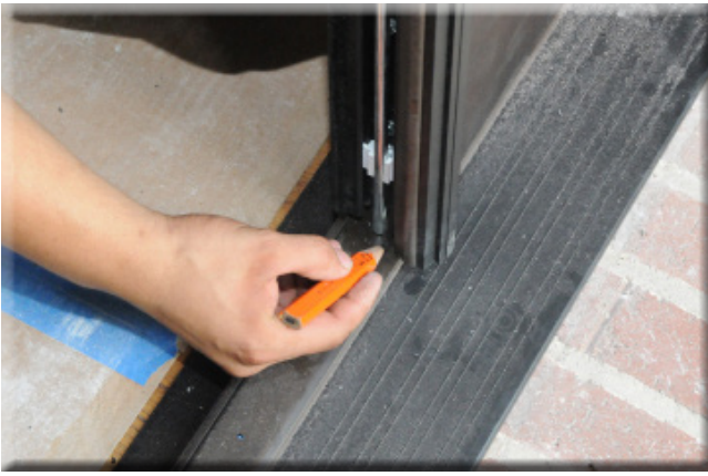
Figure 2.15.2- Make sure to apply pressure to the door while marking the bottom flush bolt position. You want this to be a tight fit so that the door seals properly.
