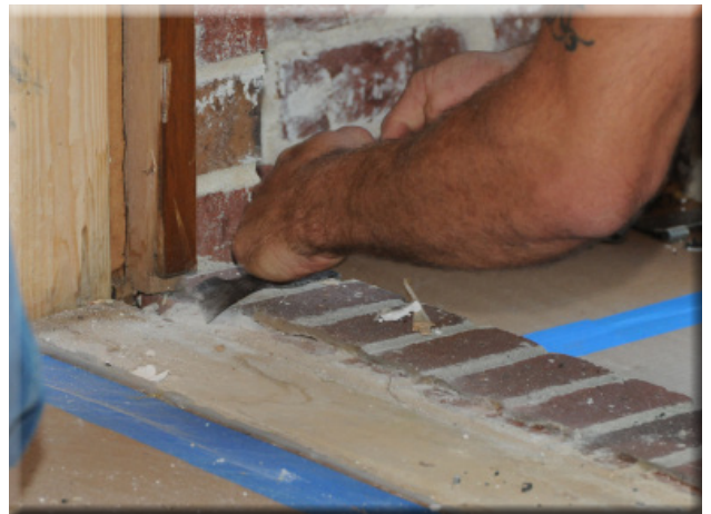
Figure 1.10- Clean the surfaces that are now exposed from the removal of the old door. A 5 in 1 scraper works well here.
