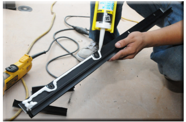
Figure 2.16- Use acrylic caulk instead of silicone here. It will be easier to adjust the sweep in the future if needed.
