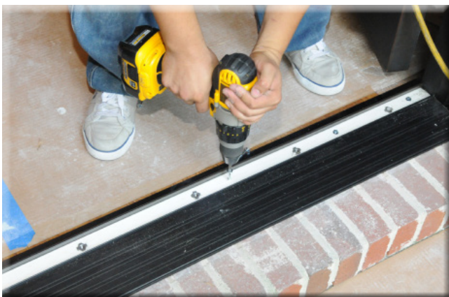
Figure 2.14.2- Secure the threshold using 2" wood screws.
