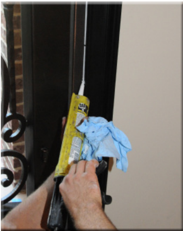
Figure 3.1- Using white caulk is okay. You will be painting it to match the door.
