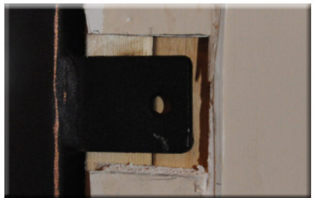
Figure 2.5- Tab should sit against studs.
