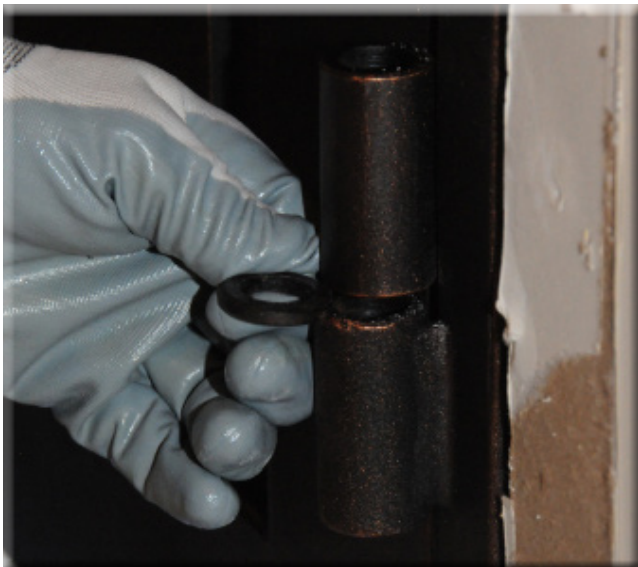
Figure 2.10- The hinge bearing must be installed at this step. The door will not align properly without it.
