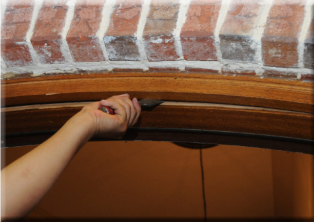
Figure 1.7- If the brick mold is in good condition, leave it. It can be painted to match the door.
