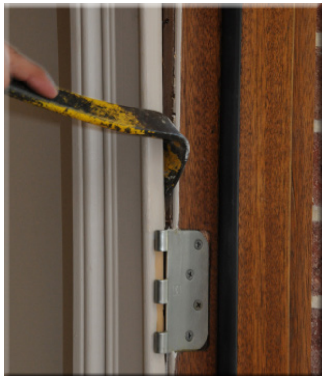
Figure 1.3- A pry bar works nicely here. Be very careful, though, as this piece of trim will be reused in most cases.
