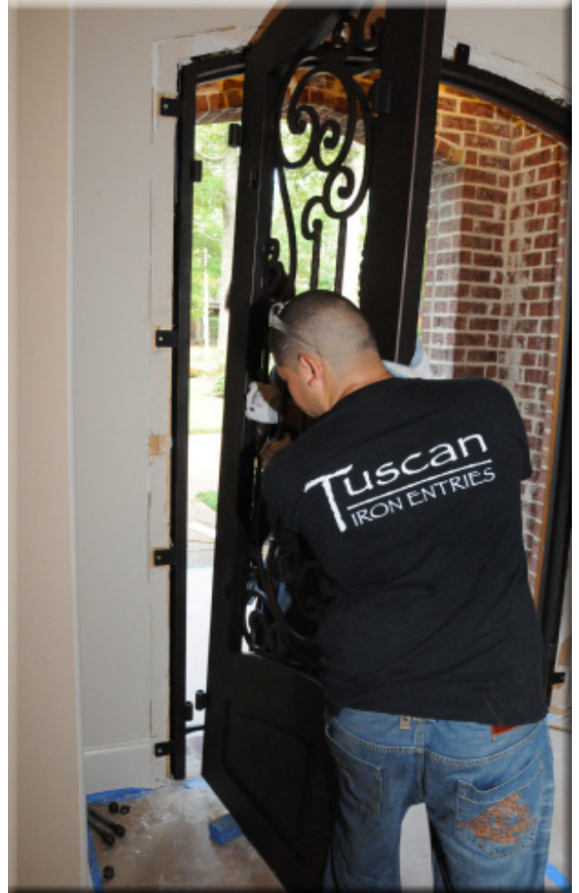
Figure 2.8- The block will help keep the door at the correct level while you are trying to set the hinge pins.
